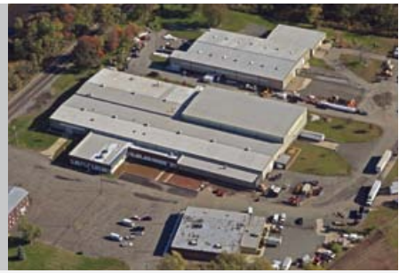
The new PARO facility now holds manufacturing, installation, final paint, as well as ample office space
