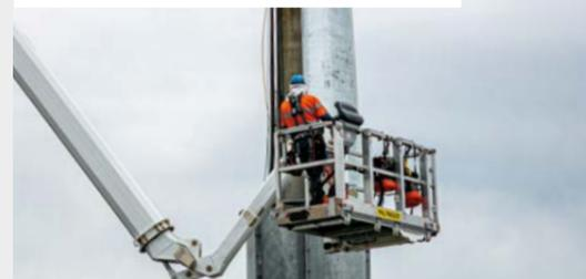
Working on telecommunication masts and on power lines requires particularly strong safety features. Overhead lines, for instance, must be disconnected if the work platform is not strongly insulated. For live power lines up to 1000 V, a double-insulated basket already provides excellent protection.
